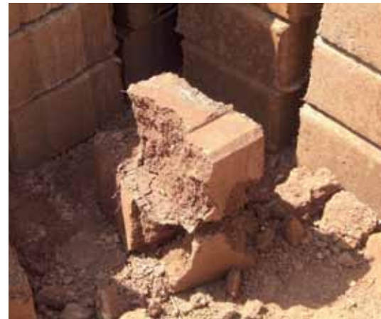
Top photo: The bricks made of local earth are not weatherproof. Often enough, a series of tropical rainfalls can cause the houses to collapse. Centre and bottom photos: The mud bricks were mostly made by hand – from cutting up the plant material with shears or a maize mill to preparing the mixture. The final process was performed with a two-pivot block machine.
