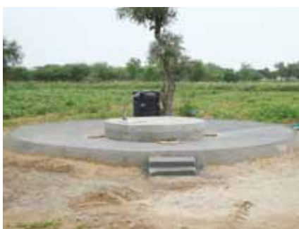
The catchment area of the rainwater harvesting pond is also utilised for drying and threshing crops.
