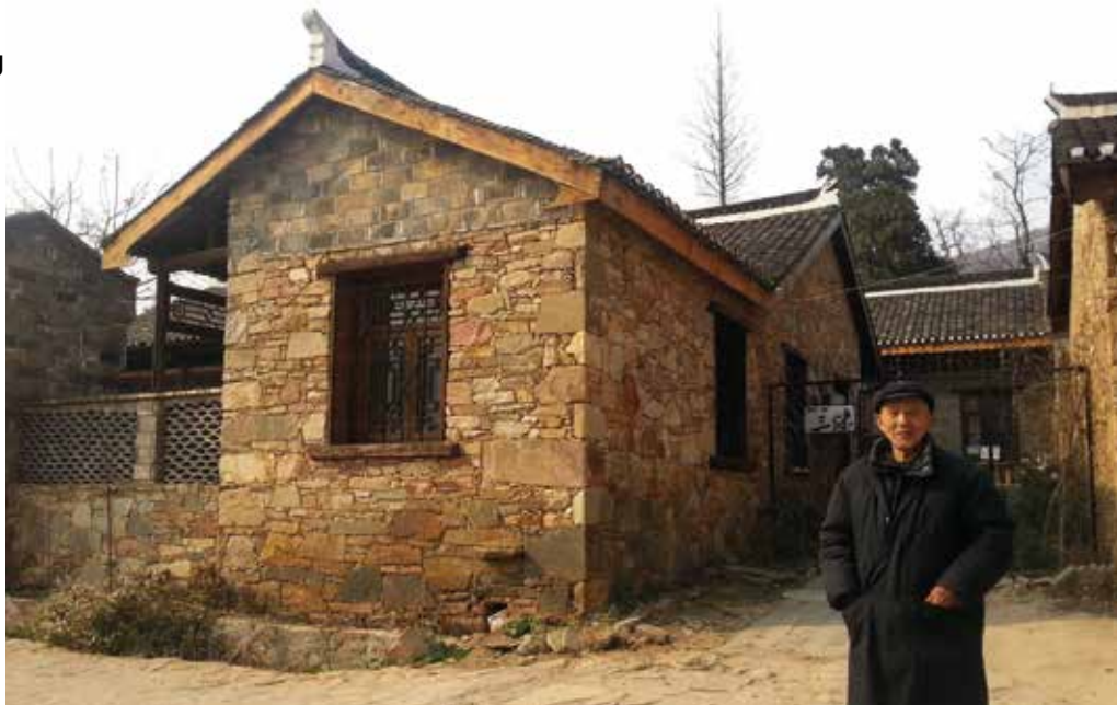
Retaining the original building fabric is an integral element of the green Happiness Village project.
