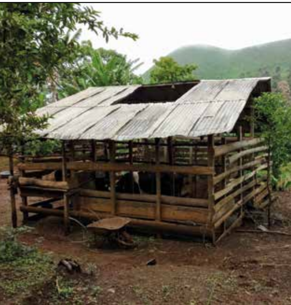
A cow farm built as per Heifer International Project guidelines.
