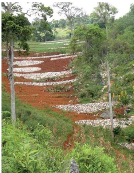
Erosion control measures to improve watershed management.
