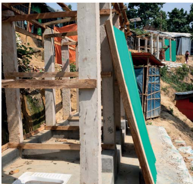
Forty latrine blocks of five to eight cabins, each connected to twelve sets of biogas plants with a kitchen, were installed.
