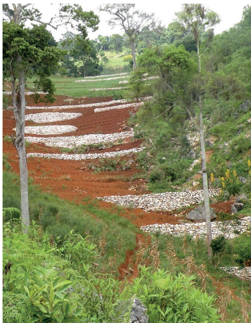
Erosion control measures to improve watershed management.
