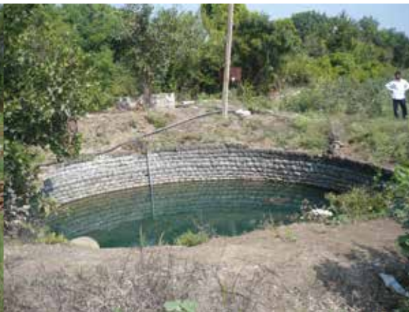
Ex-situ RWHM: a rainwater storage tank for dry season irrigation in India.
