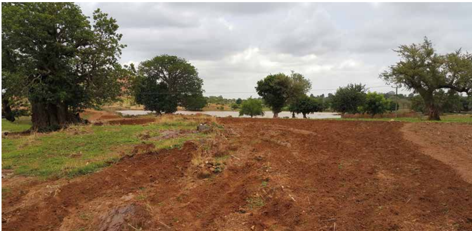
Ex-situ RWHM: a small reservoir for dry season irrigation and other purposes in Ghana.
