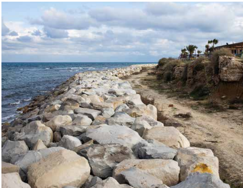
Coastal protection project close to Hergla and Hammam Sousse. Ancient roman settlements are protected from further erosion via coastal walls and groynes.
