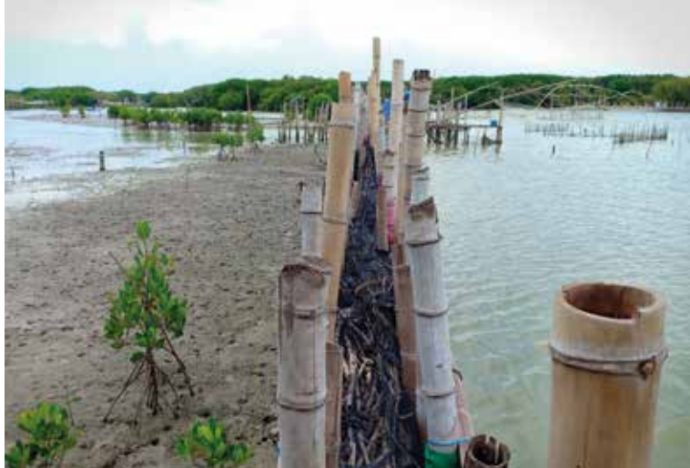
In muddy coasts, permeable dams trap sediments and gradually create habitat for natural mangrove rehabilitation.
