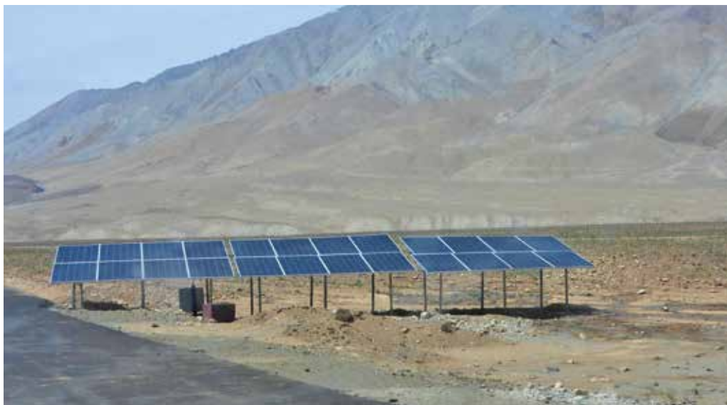
Solar energy is used to irrigate the tree saplings with ground water in early summer, when glacier-melt is not available.
