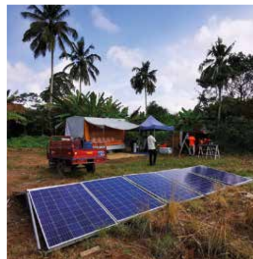
The mobile pressing unit is powered with solar energy.
